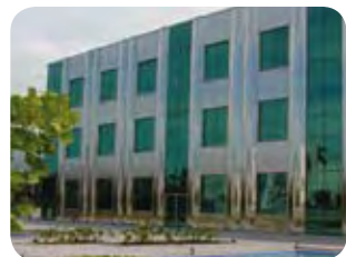
Partially 444 building cladding, Brazil.
