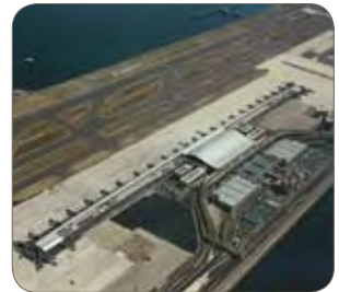
Grade SUS 447J1, Kansai Airport terminal building (architect Renzo Piano), JSSA, Osaka, Japan
