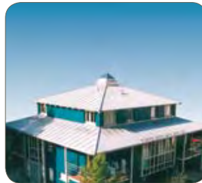
Grade 1.4510/430Ti (standing-seam technique), Ugine & Alz, Germany.
