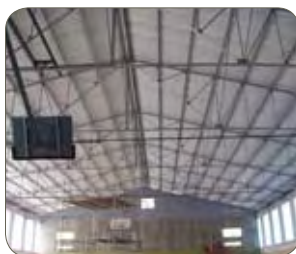
Roof-support: a potential application for ferritics.
