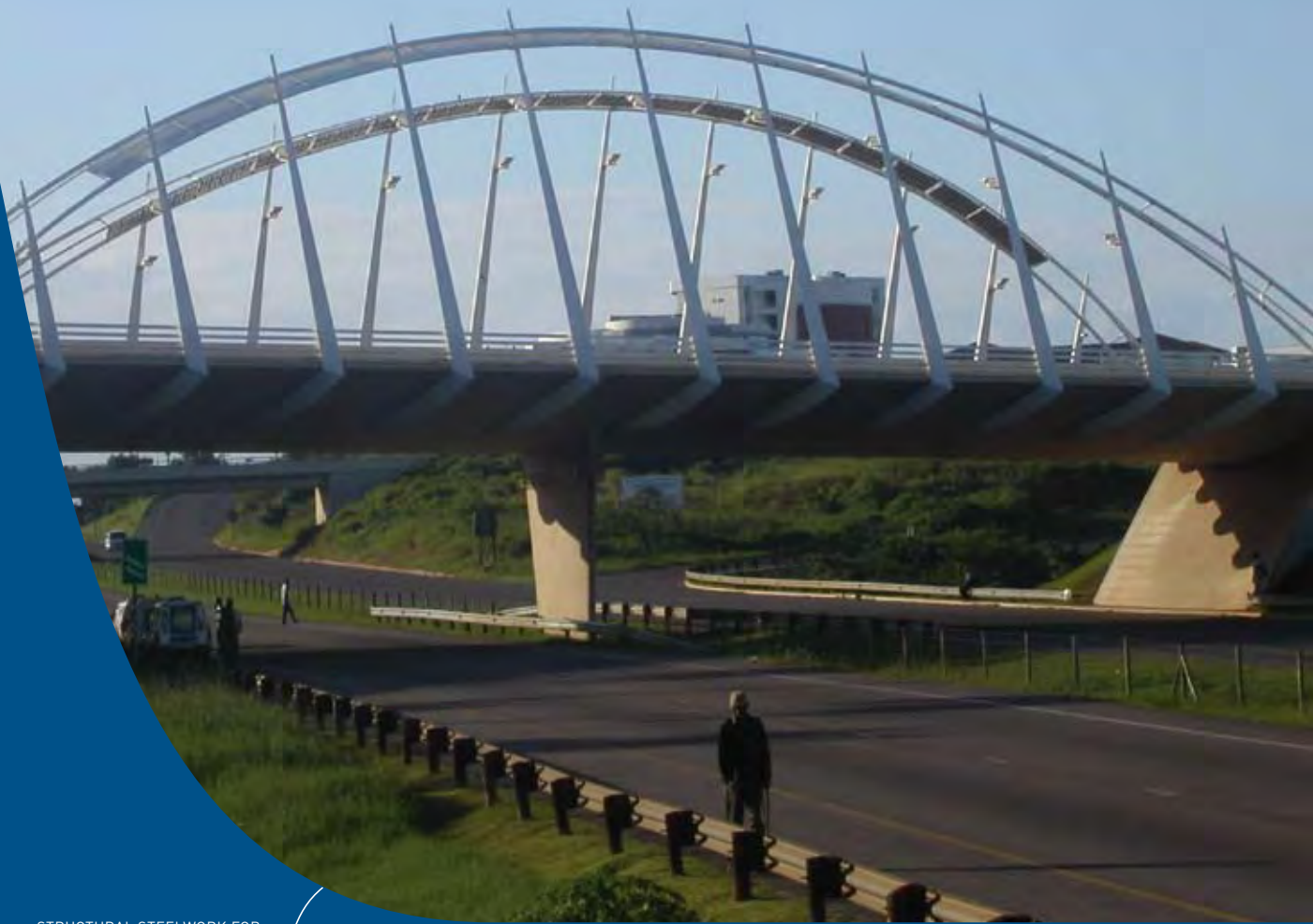
STRUCTURAL STEELWORK FOR HIGHWAY BRIDGE IN DURBAN, SOUTH AFRICA, OF PAINTED FERRITIC STAINLESS STEEL.
