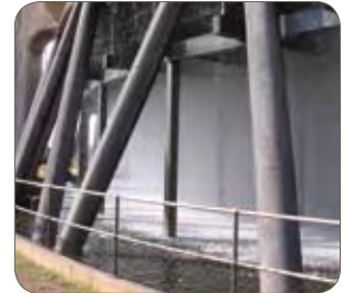
Grade 1.4003/ 410, X-grid cooling tower packing, S.Africa
