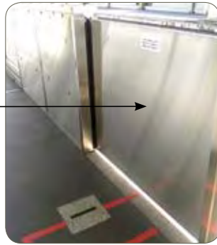
Railway station safety barrier, in SUS430JL, Japan.
