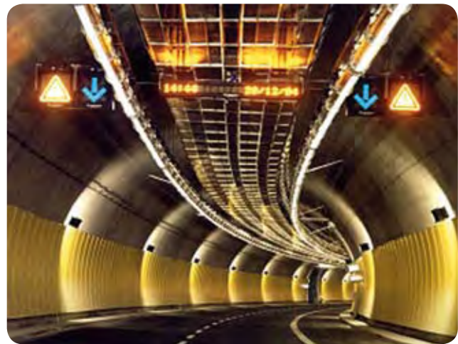
Cladding panels, in coated grade 430, Italy.
