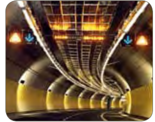
Grade 1.4016/430, painted, Monte Mario Tunnel, Centro Inox, Italy
